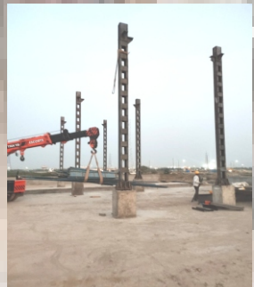
KILBURN CHEMICALS SHED FABRICATION
